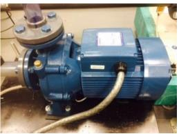
Fig. 2. Centrifugal pump type F32/200AH.
