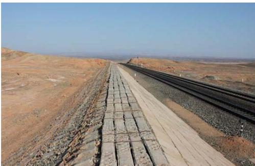
**Fig. 1. Earth embankment type windbreak wall along the Lanzhou-Xinjiang railway.**
