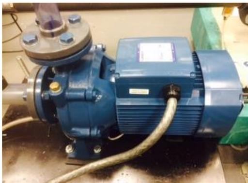
**Fig. 2. Centrifugal pump type F32/200AH.**
